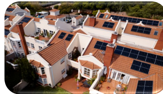
Apartment complex in Randburg
