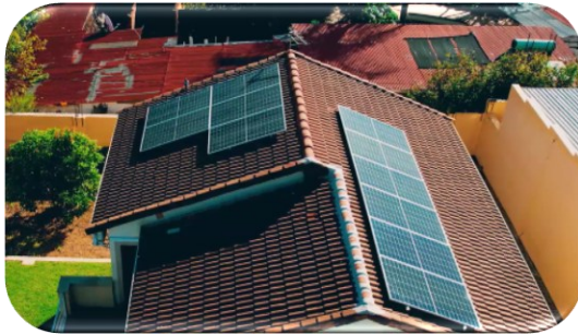
Residential installation in Johannesburg
